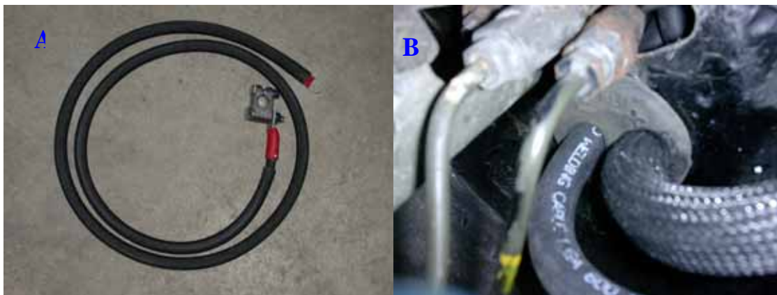
Image 19 - A. Positive battery cable. B. Negative and positive battery cables going through the firewall grommet.
