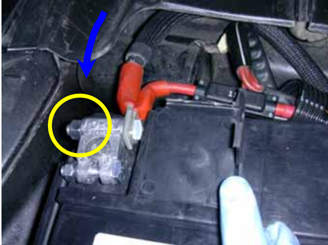
Image 24 - Bolting the positive cables to the battery post
